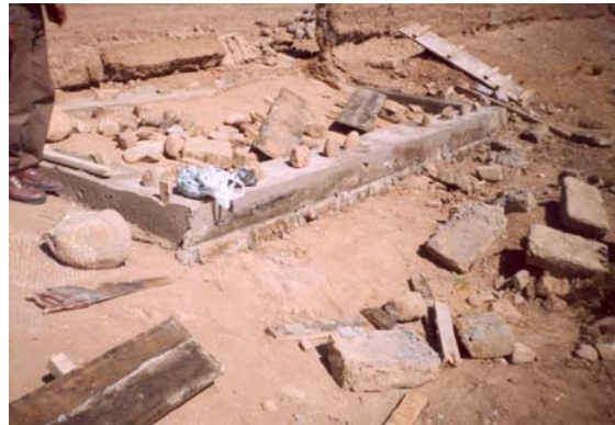
Building the latrines at the Elizardo Perez School. Delivery of material for the building of the latrines. The outline of the base is in the foreground (upper left). Forming the foundation (upper right). The latrines start to take shape as a few layers of brick and mortar are finished (right).
