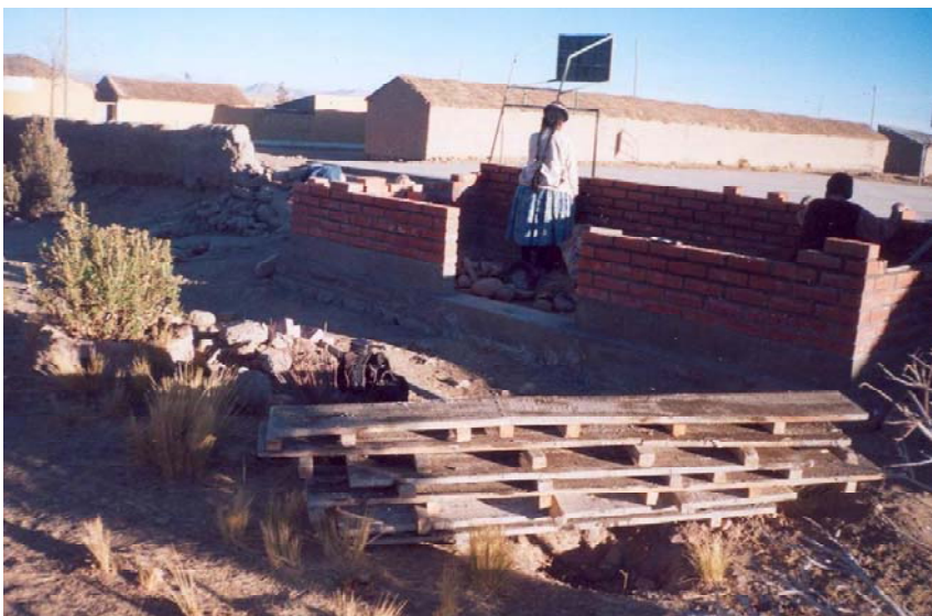
Building the latrines at the Elizardo Perez School. Delivery of material for the building of the latrines. The outline of the base is in the foreground (upper left). Forming the foundation (upper right). The latrines start to take shape as a few layers of brick and mortar are finished (right).
