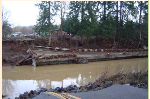
Chandler Road Bridge in Chehalis River
